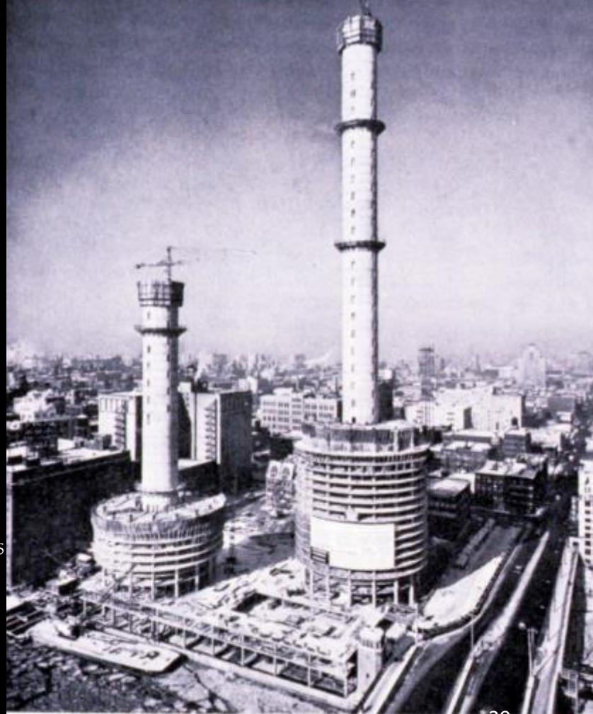
FIGURE 7.18 Marina Towers in Chicago during construction.
